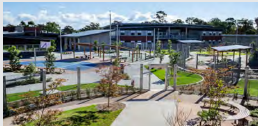
Dillwynia Correctional Centre | Security & communications design | NSW | 2018-2020
