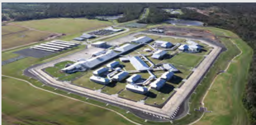
Southern QLD Correctional Precinct | State electronic security & communications adviser | QLD | 2019-2022
