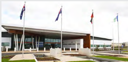
Ravenhall Correctional Centre PPP | Security design & independent reviewer | VIC | 2014-2017
