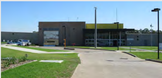
Cessnock maximum security 330-bed expansion | Security design | NSW | 2017-2019
